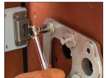
4 - Secure with 1/2" Socket Wrench
